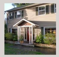
Process – Set project plan in motion and established budget. Designed floor layout and procured engineering plans and permits. Dug basement out, set foundation and finished. Subcontracted plumbing and electrical. Constructed 2nd floor framing in backyard. Demoed roof, added second level by sections and Installed attic trusses.
